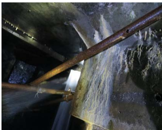
Heavy Flow Through a Drain Pipe in Intermediate Gallery at El 68.27m - Sardar Sarovar Dam
