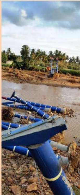
Washed away Cable Bridge on MALAPRABHA River at K Junipet, Karnataka
