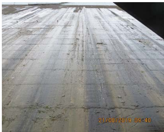
Leakage at Downstream Face of Non-Overflow Blocks- Sardar Sarovar Dam
