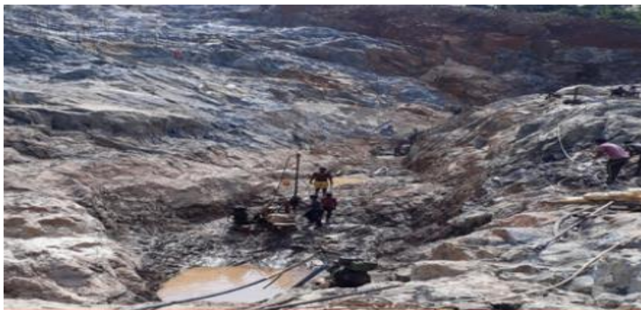
Shear zone in the foundation of the Non Over Flow portion
