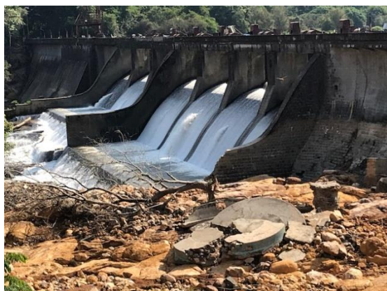
Downstream view of Poringalkuthu dam, showing damaged left training wall as well as damaged dam top road near left bank portion, and scoured dam toe during August 2018 Kerala flood
