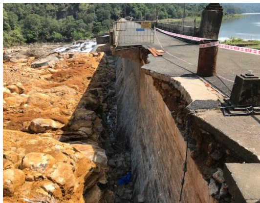
Downstream view of Poringalkuthu dam, showing damaged left training wall as well as damaged dam top road near left bank portion, and scoured dam toe during August 2018 Kerala flood
