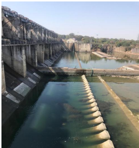
Energy Dissipation Arrangement of Ravisankar Sagar Dam
